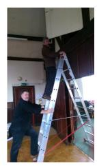
Move the ladder as close to the doorway as possible and raise the extension so that it projects into the doorway and ensure it is fixed in place. Ascend the ladder and step into the loft space using the safety handle highlighted.
